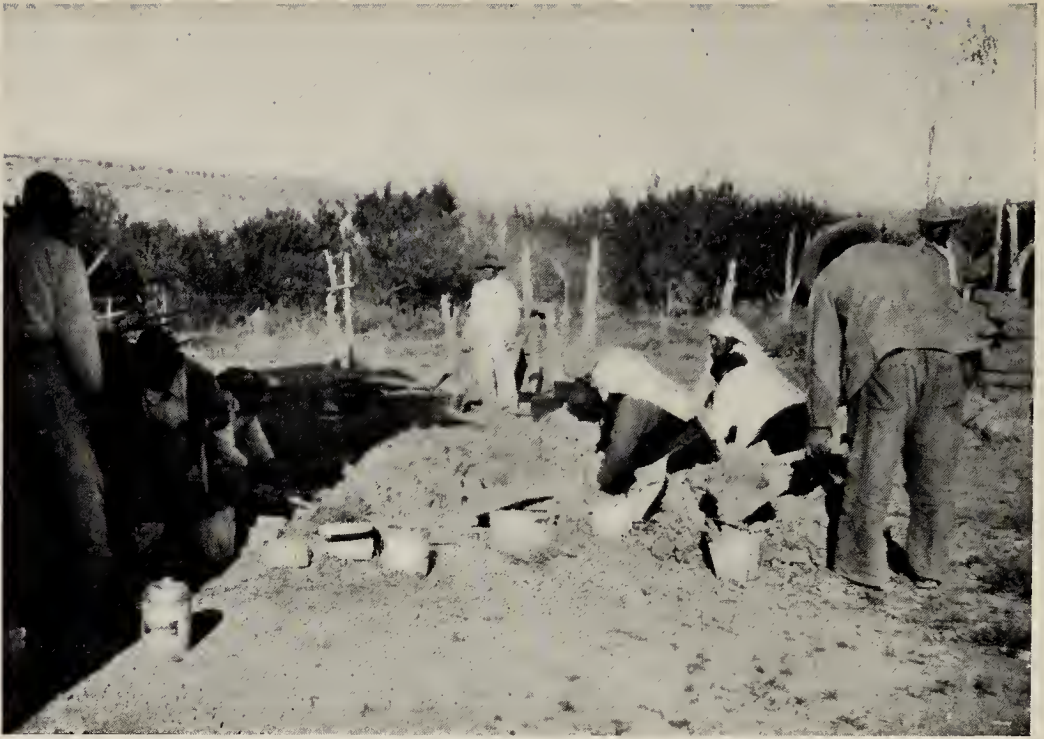
BUILDING THE CHURCH AT CASA BLANCA, N. M. The Laguna Women helped their Men in the Building
